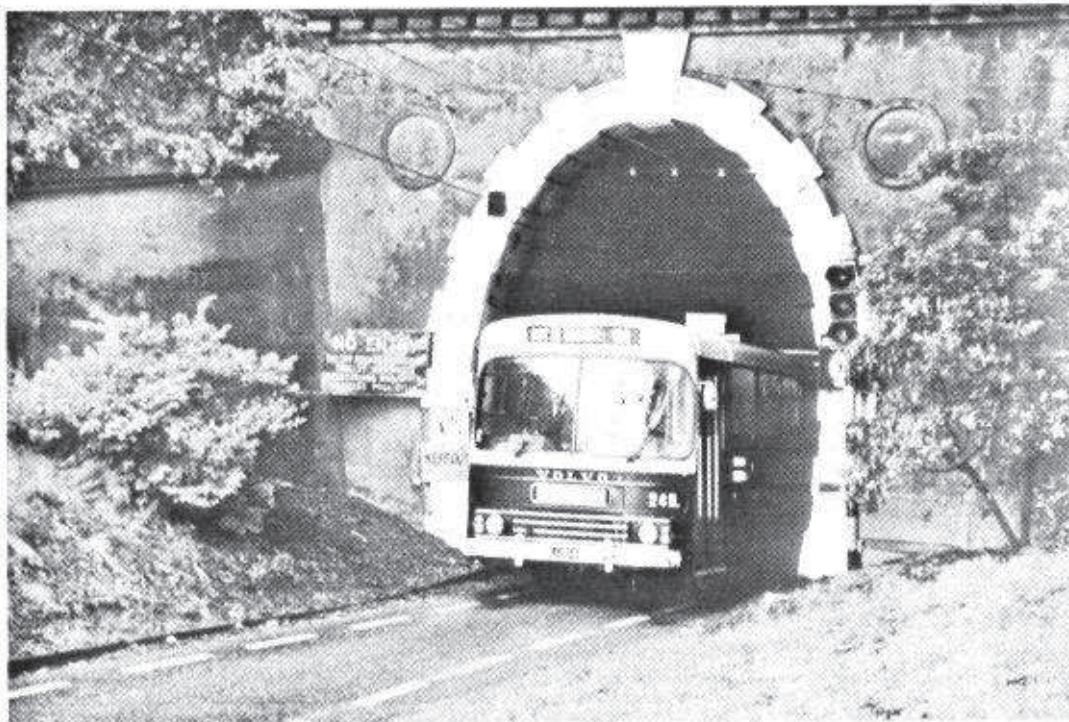
Volvo trolley bus 249 emerging from the Haitatai bus tunnel. Photograph: Les Stewart.
