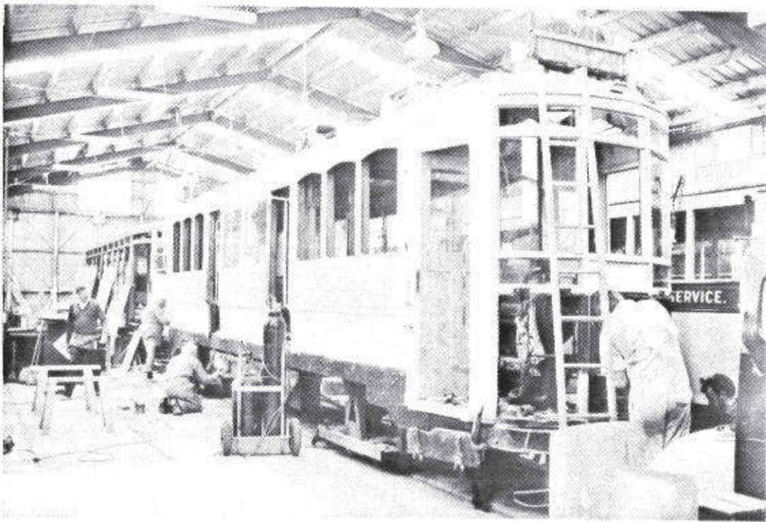
Tram 159 under restoration in November 1989. Photograph: Les Stewart.
